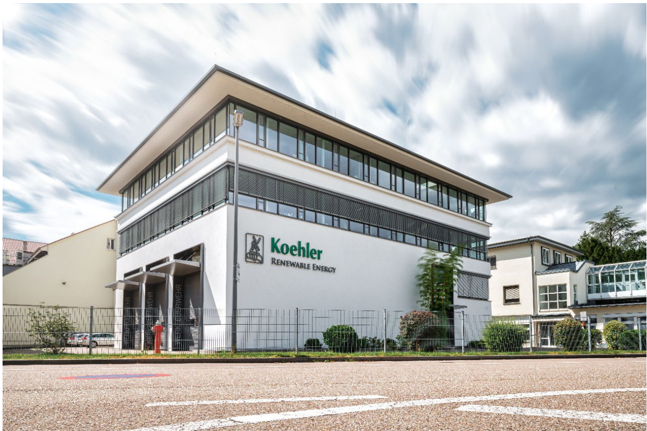
Figure: The foundation of Koehler Renewable Energy in 2012 was accompanied by a new office complex in Oberkirch / Image rights: Koehler Group
