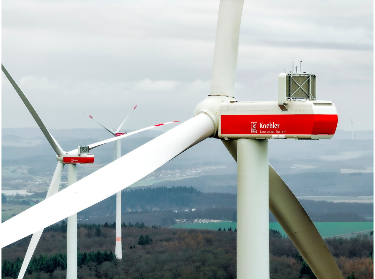
Figure: The two turbines at the Wetzlar-Blasbach wind farm are now supplying the Koehler Group with electricity generated by wind power for the first time in Germany. / Source: Koehler Group
